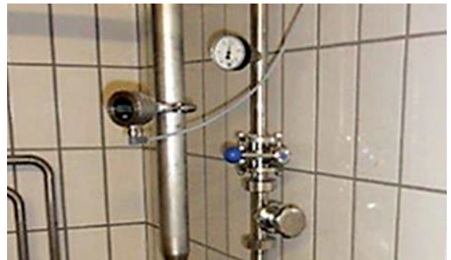
GTL 737 monitors the beer temperature of a cooling system for the keg dispenser
